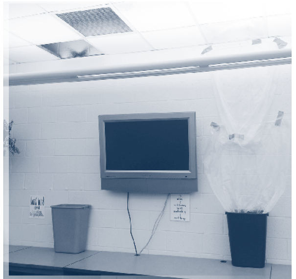
In the Pashley Elementary School library, staff place garbage pails on tables and tape plastic bags to the walls to catch water dripping from the ceiling. In other areas throughout the library the ceiling tiles, built-in counters, and walls are stained and damaged from repeated leaks. The carpets are worn and separating at the seams from overuse. The library renovations being proposed would include repairing the leaking roof, replacing carpeting, and installing new windows and air conditioning.
