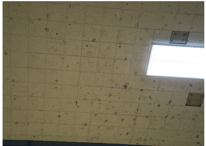
The high school's aged, disintegrating gym ceiling with missing and damaged tiles is in need of replacement.
